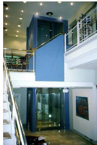
Fig. 11 and 12. The correct use of an elevator allows solving complex situations. This building that lacks space at the street level, gains access to the attic and semi-basement by a double-door elevator.
